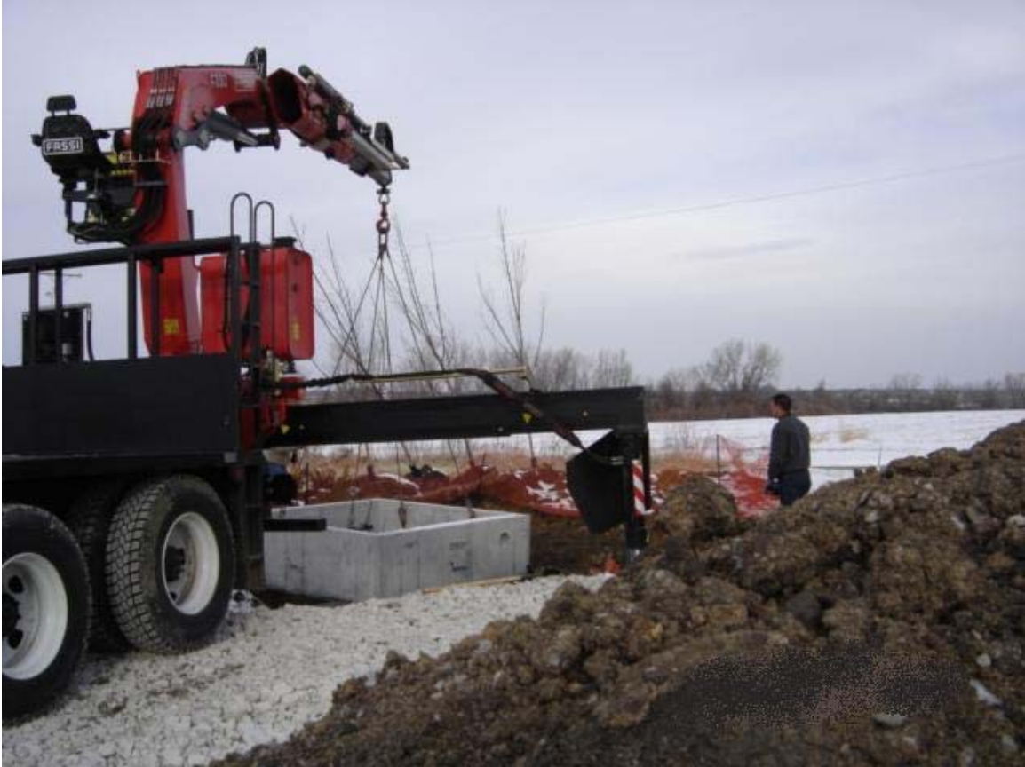
Rental Truck w/ F330 & 16,000 lb Vault
