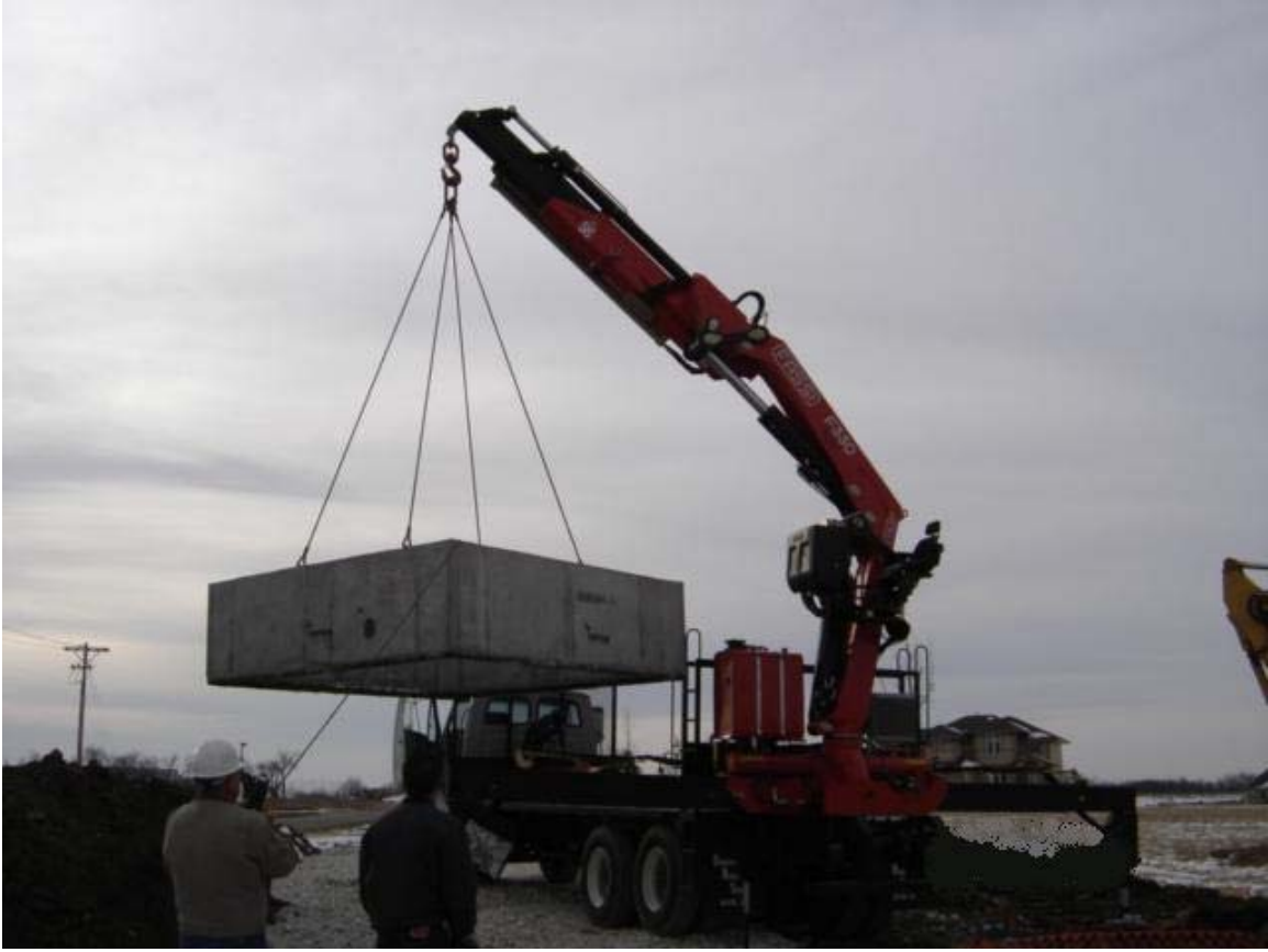
One of Our Rental Trucks w/ F330 Placing a Vault
